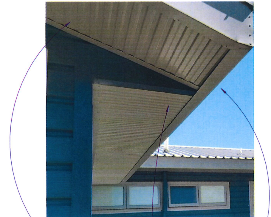
Photo C Proposed Eave Boxing In Colorbond
