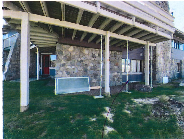
Photo B Existing Deck & Proposed Recladding
