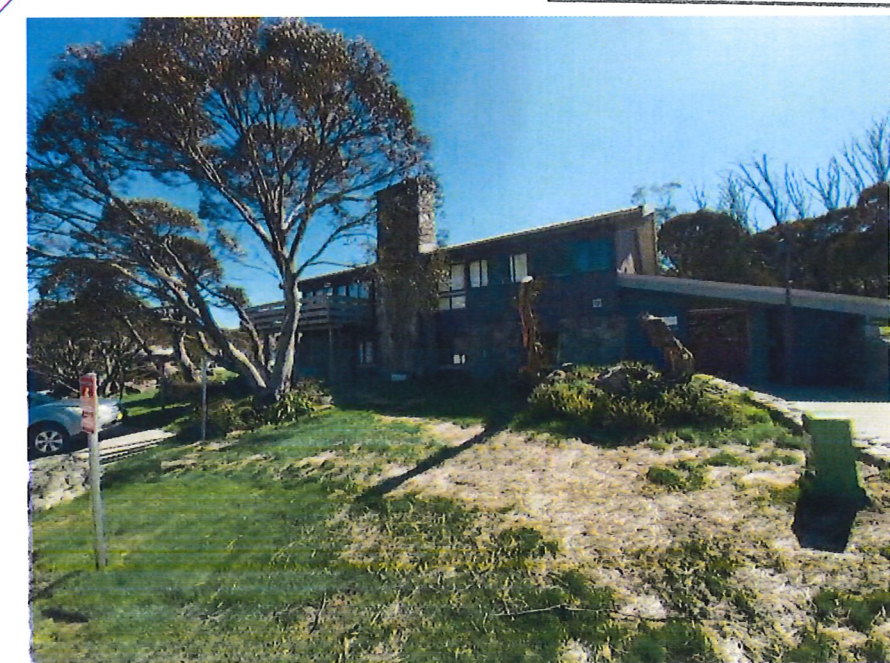
Photo B Existing Carparking
