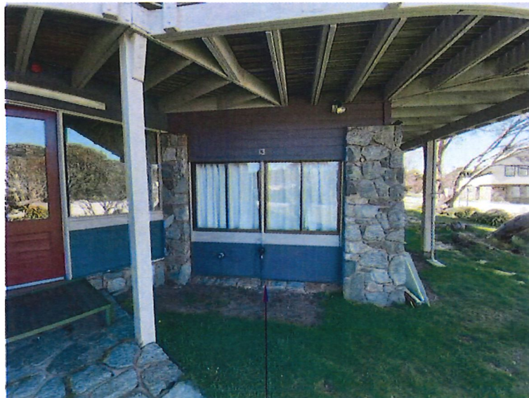
Photo A Existing Deck & Proposed Recladding
